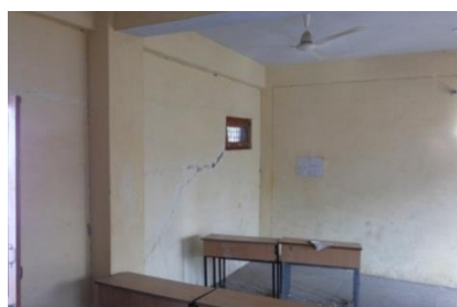
Fig.14 Incorrect ventilator placement
