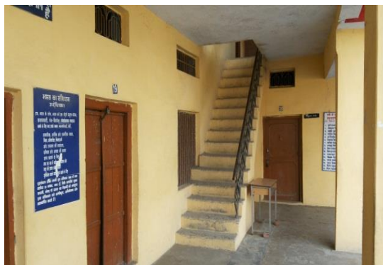
Fig.26 Number of stairs present exceeds max. limit per flight. (GSSS Chabutra)
