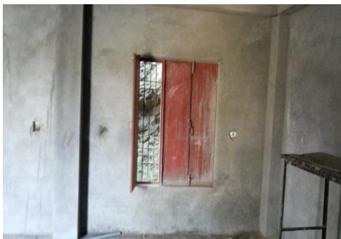
Fig.31 Steel windows inappropriate for illumination Requirement (GPS Panyala)
