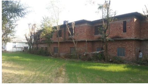
Fig. 17 Irregular wall pattern responsible for Increased wind speeds. (GSSSTal)
