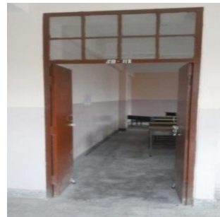
Fig.19Good example of exit (GSSS Nalti)
