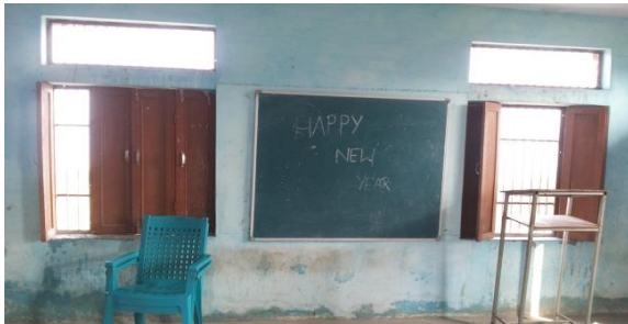
Fig.23 Wrong placement of greenboard causing glare. (GHS Bralhari)
