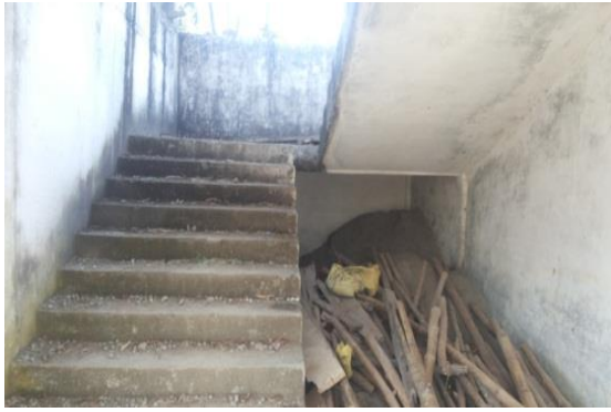
Fig.27 Handrail not installed.(GSSS Bhota)
