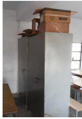
Fig.32 (a)improper placement of bookshelves makes it difficult to operate(GSSS Chabutra) (b)Unanchored Almirah(GPS Panyala) (c) Unanchored computer equipments(GSSS kot) (d) Unanchored Almirah placed in classroom (GSSS kot)
