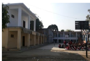
Fig.11 Irregular plan(GSSS kot) Fig.12 Vertical and plan irregularity(GSSS Tal)
