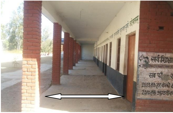
Fig.21 Corridor area limit exceeded (GSSSBhota)
