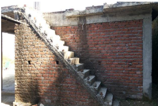
Fig.25 Open stairs not as per standards (GPSPananyala)
