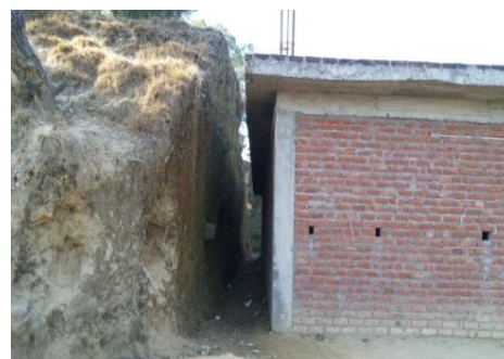
Fig.16 inappropriate distance between cut boundary slope and building wall (GPS Panyala)
