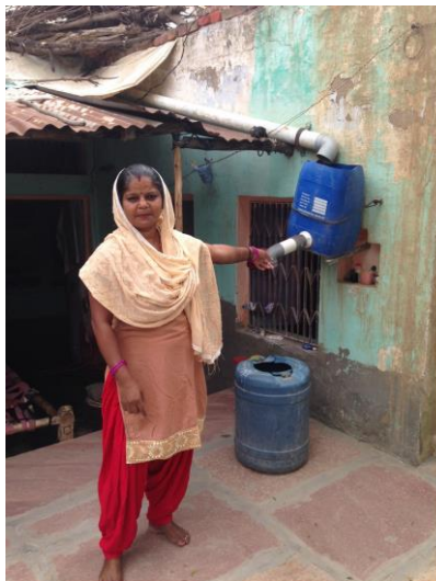
Group leader Gayatri Devi, who installed a RWH unit at her home
