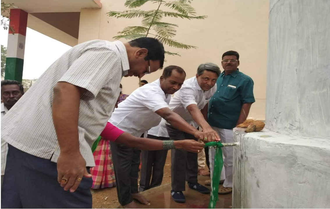
Water tank, sump, other civil works inauguration programme on 26.01.2019 with the help of donors at ZPHS (B) Gopalpet.
